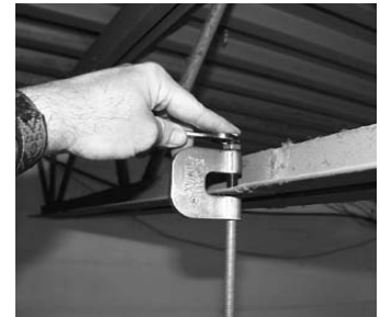
Fig. 2 Attaching Beam clamp to the building structure
