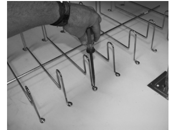
Fig. 1 Attaching the 101 Series Snake Tray to the floor using CM-CA-38 anchor bolts
