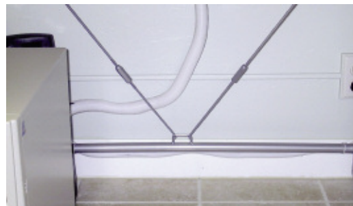
After with White 1" X 5' Wire Loom
